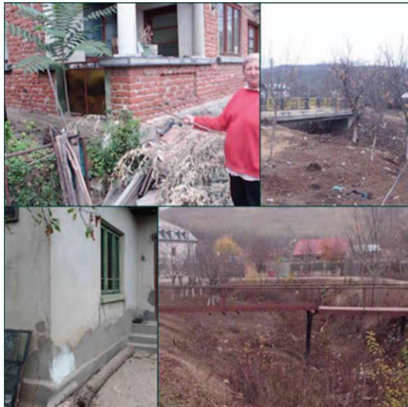
Figure 10. Images illustrating the damages after the flash flood in Lazu village (Morosanu, 2012)
