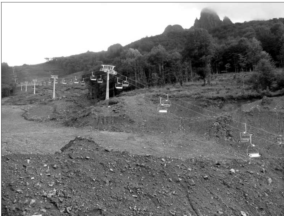
Figure 2. Photo of the degradation of the terrain caused by construction of lifts within ski centre “Babin zub” (Rubinjoni, 2008 2 )
