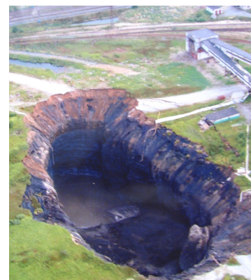
Fig. 2. Enormous collapse in Berez-niki city, Perm region (2007)
