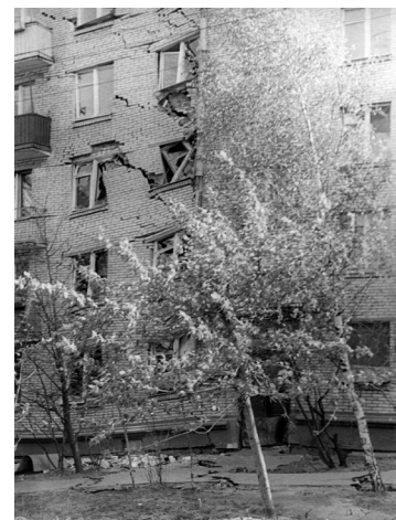
Fig. 3. View over local subsidence under residential building in Moscow (1977)
