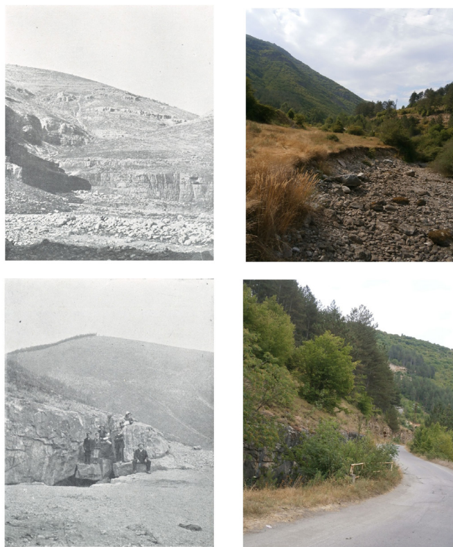
Fig. 5. Top: The area of Iskrets karst springs in 1915 and 2015. Bottom: The entrance of Dushnika Cave (876 m) near the village of Iskrets in 1915 and the same place today
