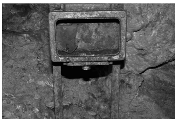
Fig. 14. Remains of a power distribution cabinet (ph. by M. Kličković)
