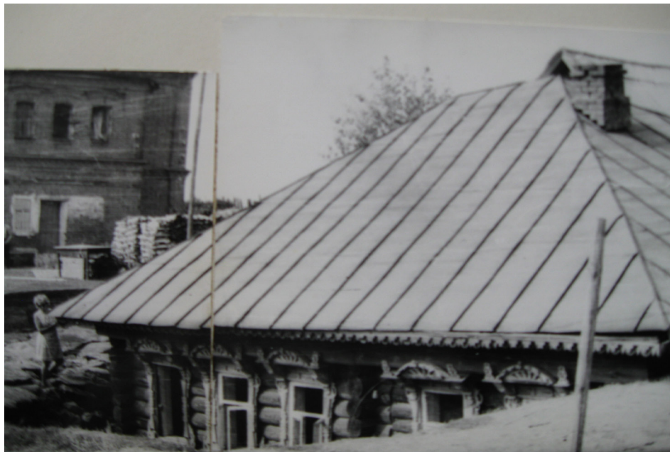
Fig. 1. Sinkhole collapse caused under residual building (Rasstrigino, Vladimir region, Russia, 1972)
