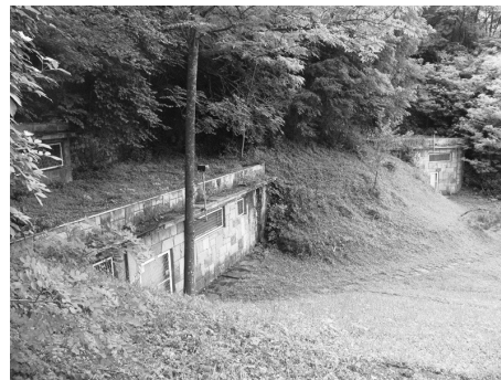
Fig. 3. Studena water supply source: spring captures ( http://www.jkpnaiissus.co.rs )
